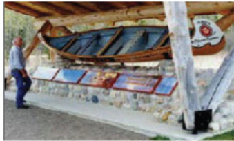
Canoe Pavilion - RMH National Historic Site, 1992
